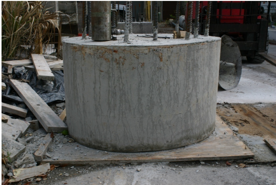
Figure A.27. Shaft 18, water shaft after pressure washing.
