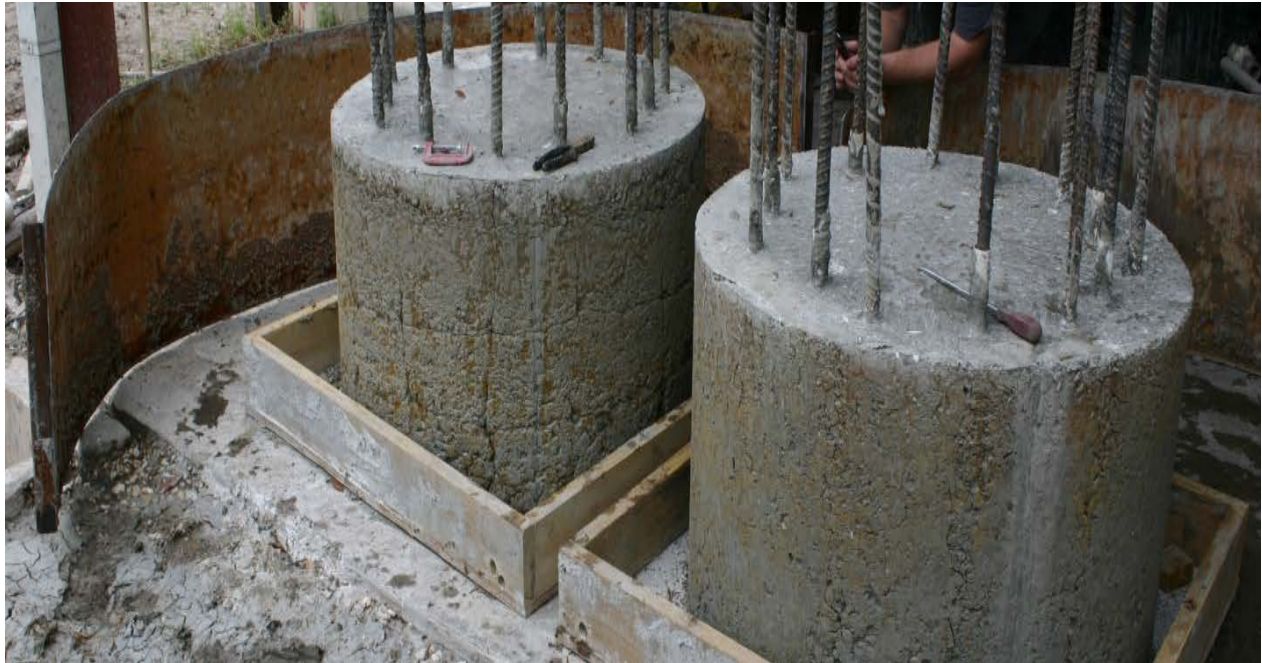
Figure 4.7. Illustrates the 90 second (left) and 40 second shaft (right) from placement one following form removal.
