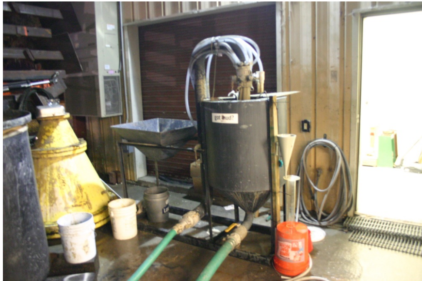
Figure A.9. Re-circulating mineral slurry prior to placement in form.
