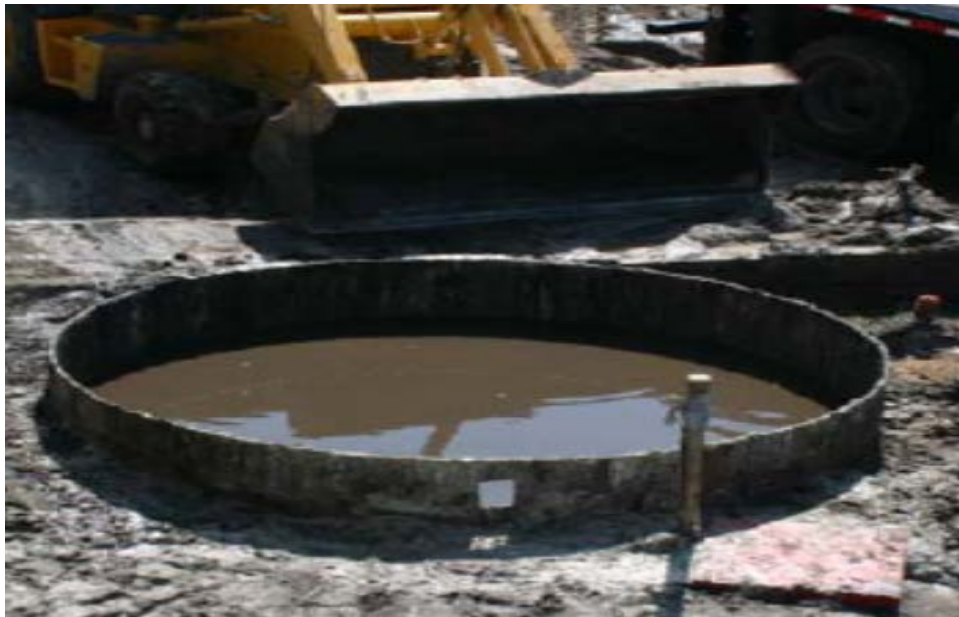
Figure 2.2. Temporary surface casing providing containment for slurry.
