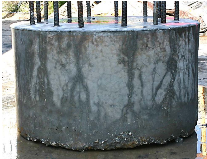
Figure A.15. Shaft 6 (water) after pressure washing.
