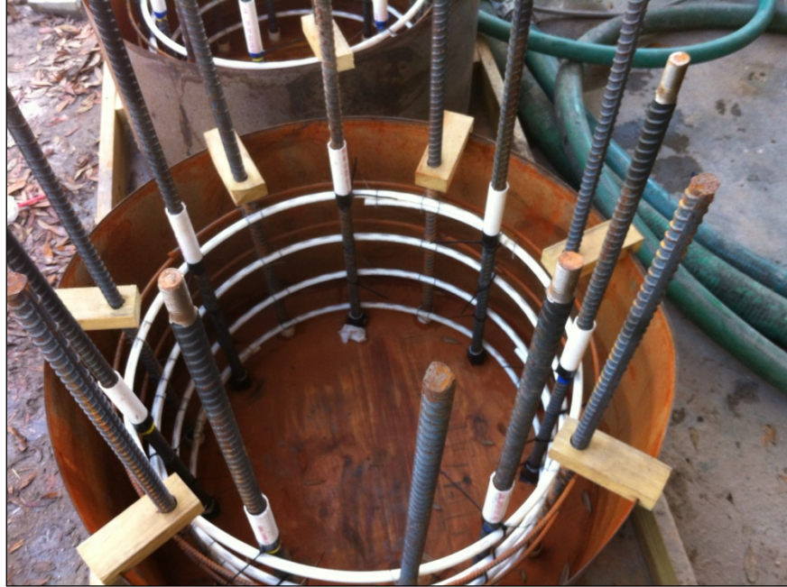
Figure A.6. Final reinforcement configuration prior to slurry placement.
