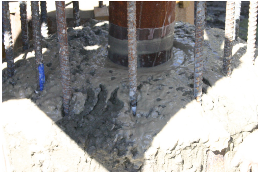
Figure A.11. Placing concrete for shaft 2, 90 sec/qt mineral slurry.
