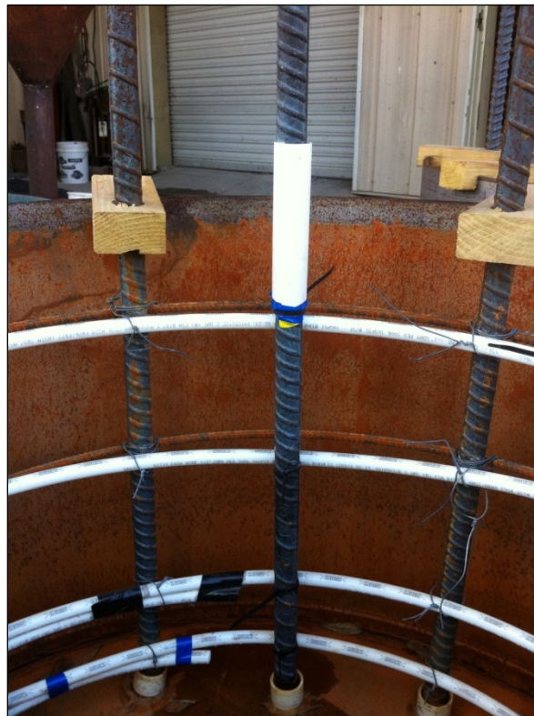
Figure A.7. Typical de-bonding for reinforcement.
