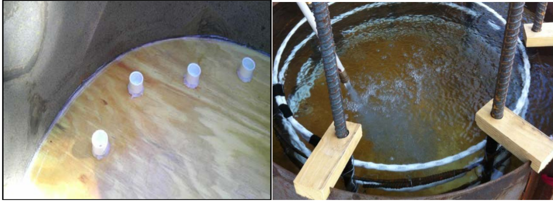
Figure 3.5. Silicon to seal form (left), water testing to ensure water tight seal (right).
