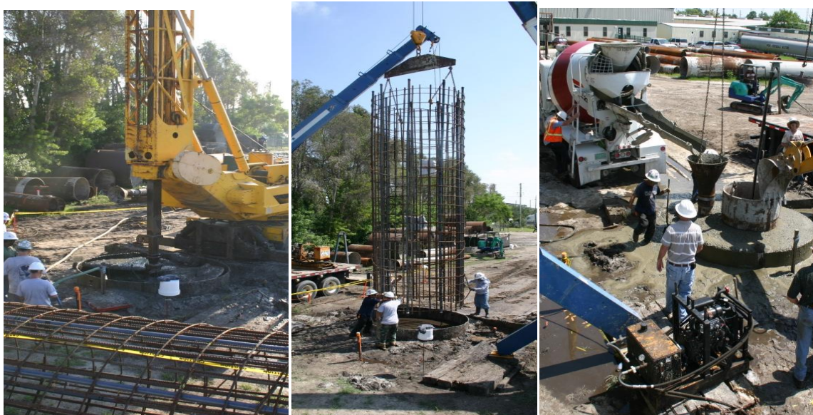
Figure 1.1. Shaft construction: excavation (left), cage placement (center) and concreting (right)
