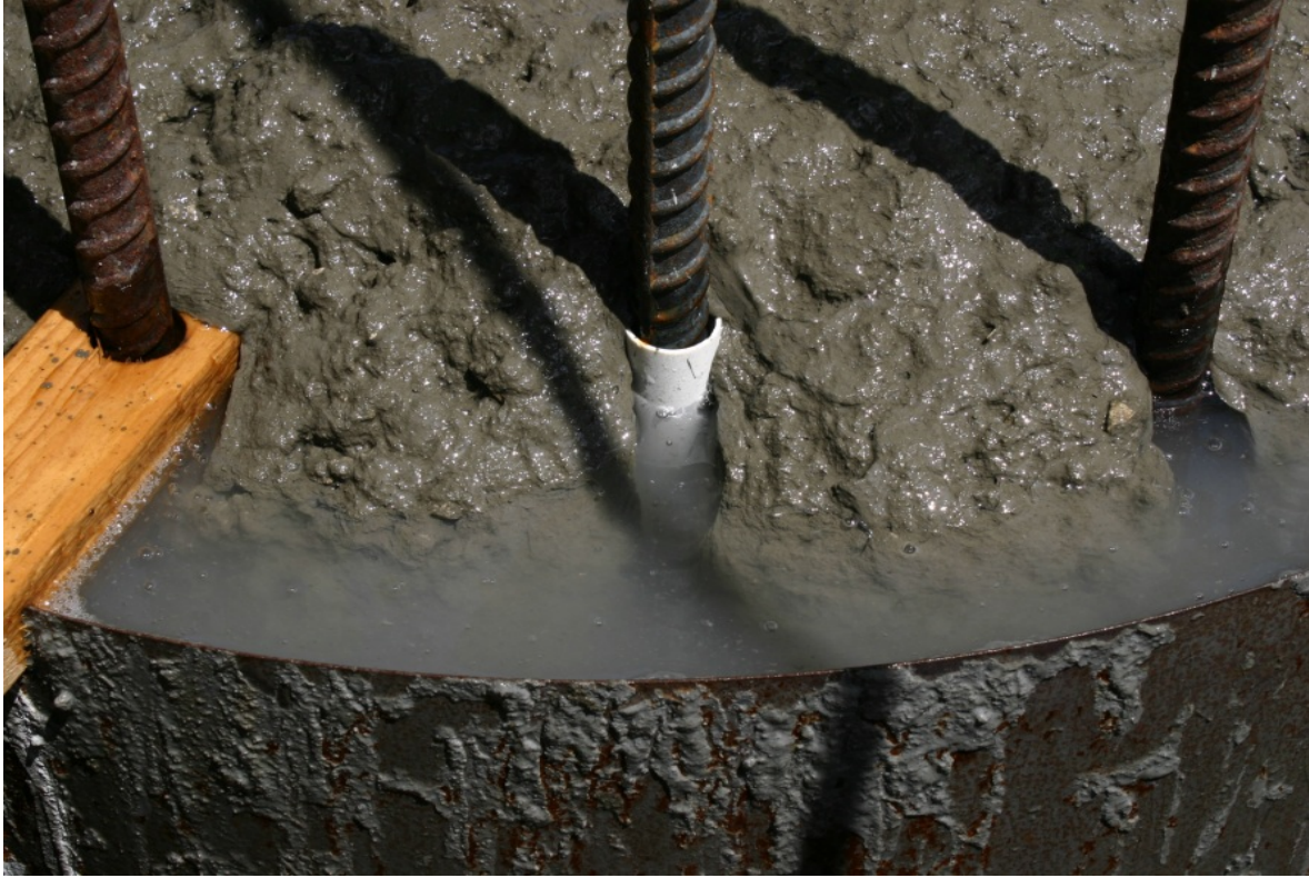
Figure 5.13. Flow of concrete around reinforcement during placement of 60 sec/qt polymer shaft.
