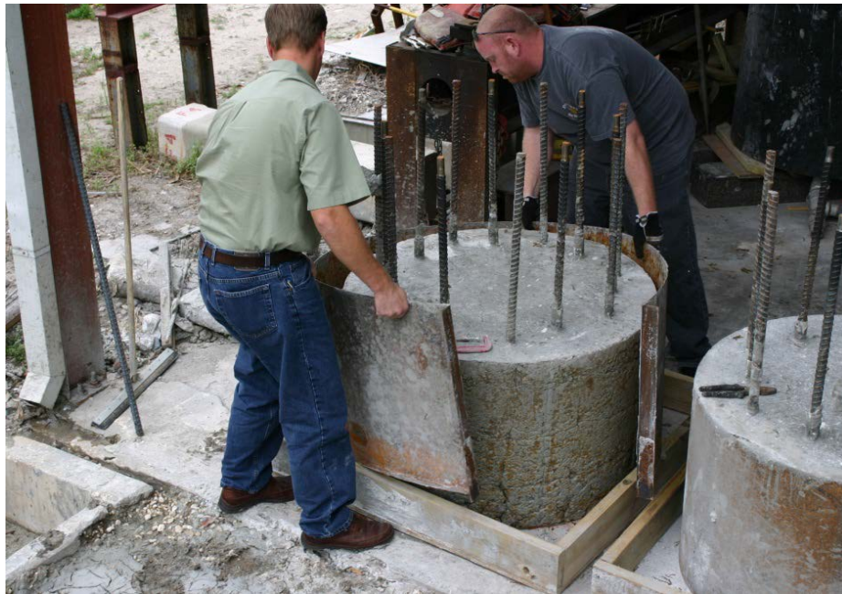
Figure 3.14. Form removal after shaft achieves suitable compressive strength.
