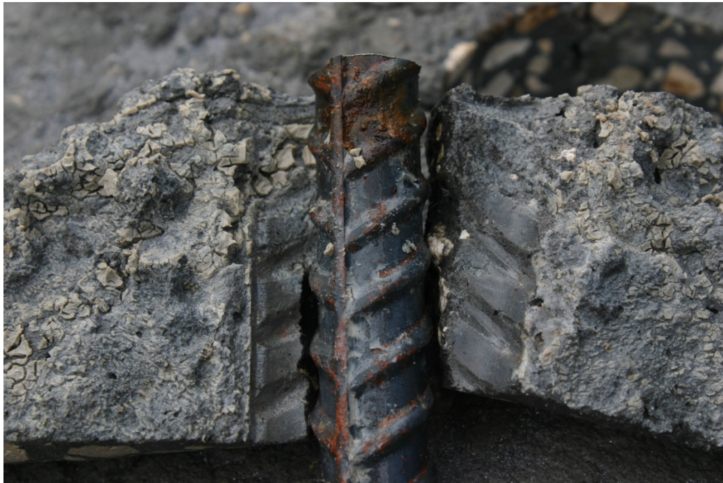
Figure 5.6. Layer of slurry encased in concrete.
