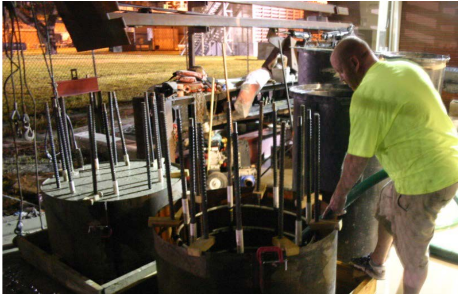
Figure 3.11. Placing mineral slurry in forms night prior to placement.
