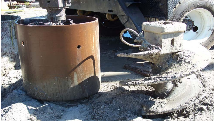
Figure 2.1. Clean out bucket(left) and flight auger (right) for shaft excavation.
