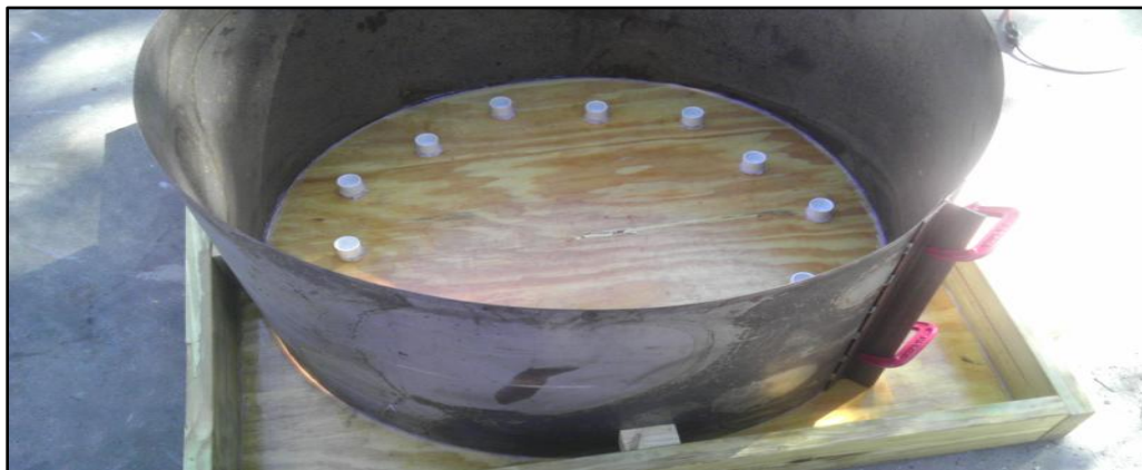
Figure 3.4. Finished form prior to placement of reinforcement.
