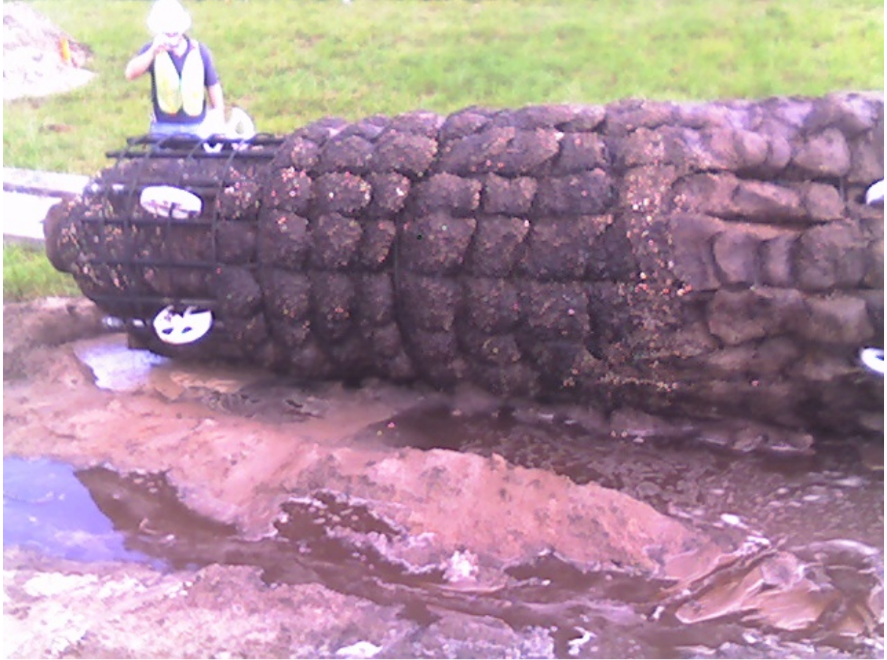
Figure 2.9. Exhumed drilled shaft displaying concrete flow issues.
