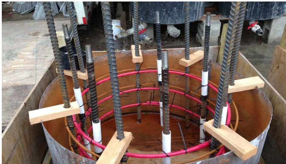
Figure 3.12. Reinforcement cage after de-bonding prior to slurry placement.
